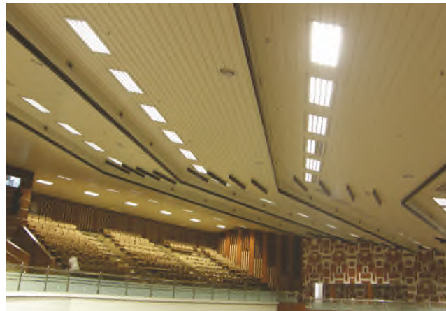
Dewan Tuanku Syed Putra, USM, Malaysia 184C (perforated/non-perforated) ceiling
