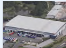
Sunflex Distribution Centre, Cannock, United Kingdom
