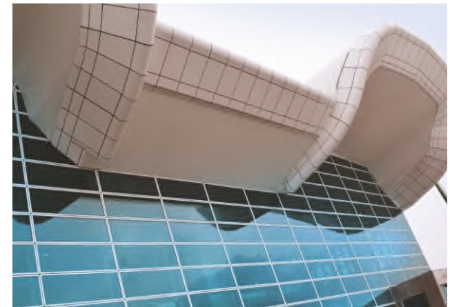
KLIA2 Malaysia 84C ceiling
