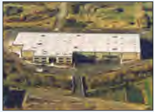
Hunter Douglas Fabrication, Renton (WA), U.S.A.
