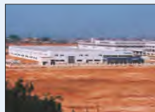
Hunter Douglas Construction Elements, Xiamen, China
