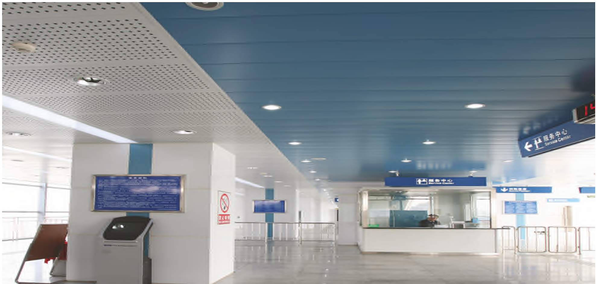
Dalian Light Rail Transit Line 3, China 300C ceiling
