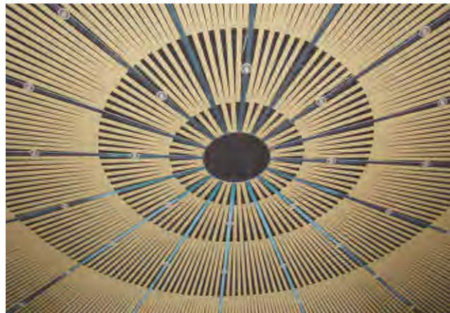
Mobifone Office Building, Ha Noi, Vietnam 84R Ceiling
