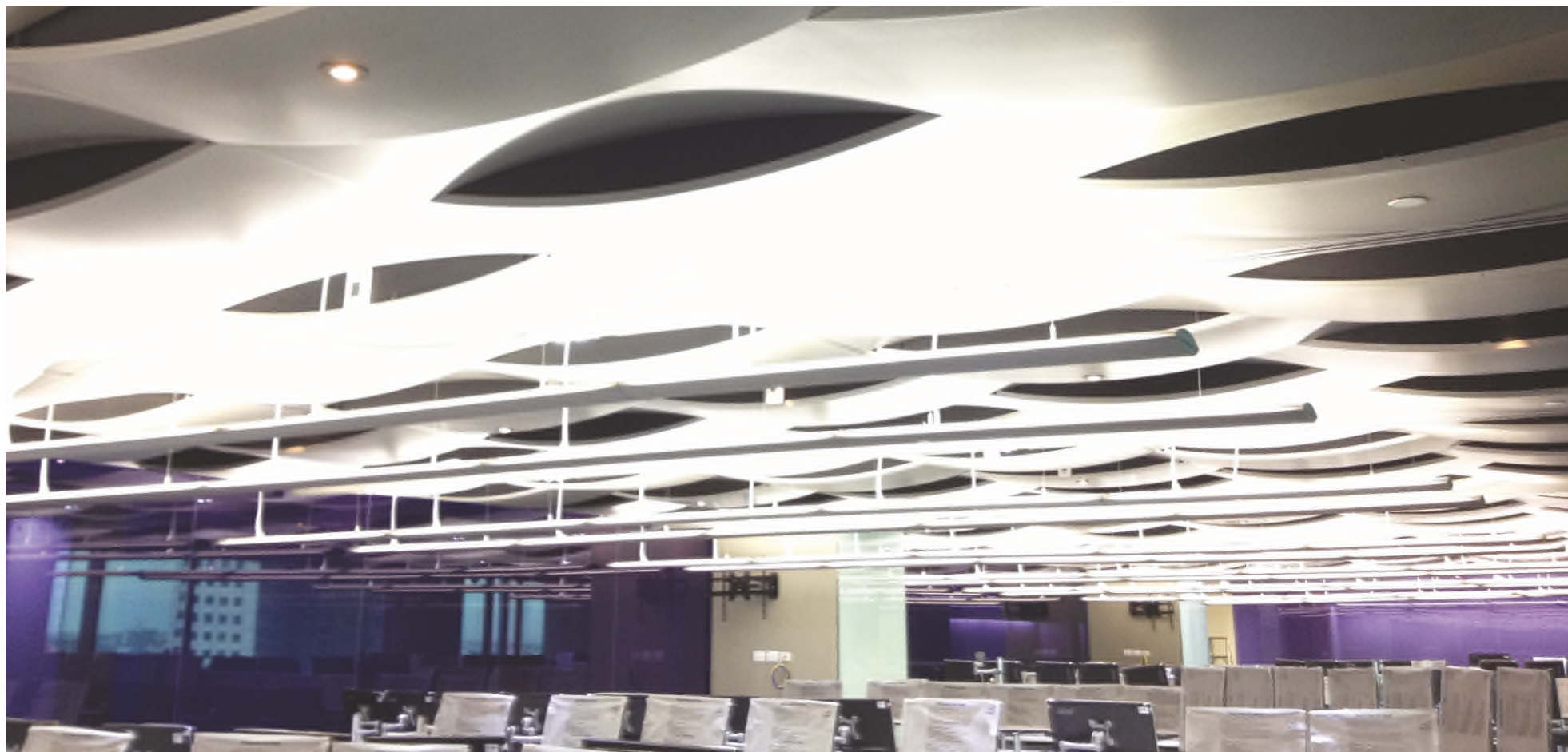
SCB Office, Thailand Honeycomb internal ceiling
