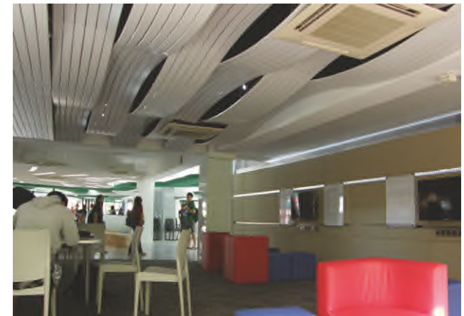
Taylor College, Malaysia 84R curve ceiling
