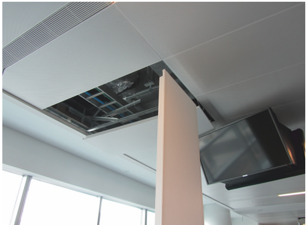
Project: JFK Terminal 4, New York
