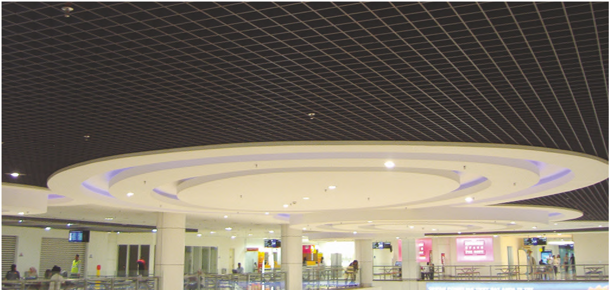
Bus Terminal Salak South, Malaysia Cell 50mm module
