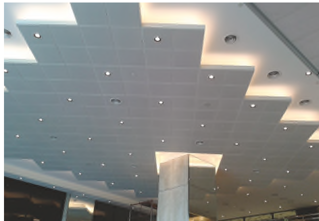
PNB Refurbishment, Malaysia Lay In Tile Perf 584mm
