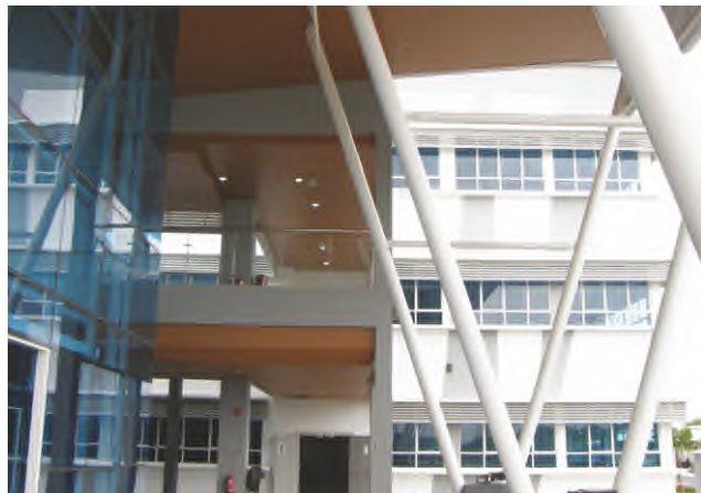
Biotect Centre, Batu Kawan, Penang, Malaysia 300C ceiling
